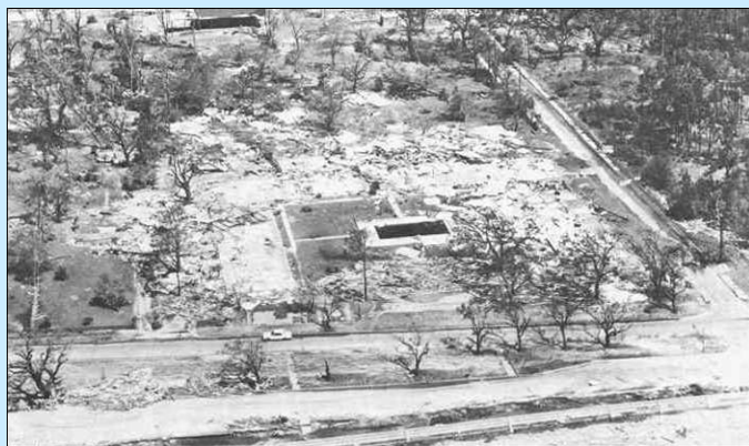
Richelieu Apartment Complex after Hurricane Camille (note pool at center)
